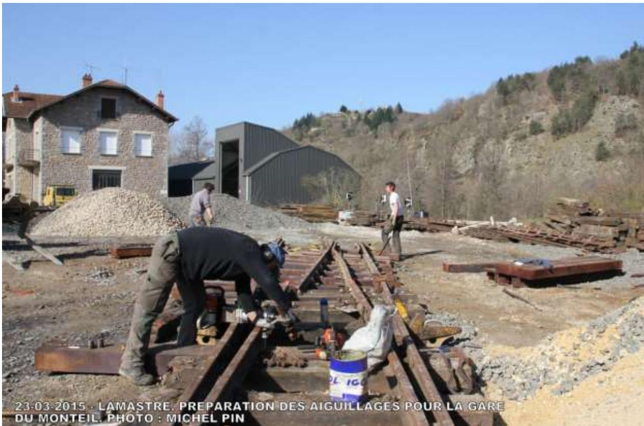
23-03-2015 - LAMASTRE. PREPARATION DES AIGUILLAGES POUR LA GARE DU MONTEIL. PHOTO : MICHEL PIN
