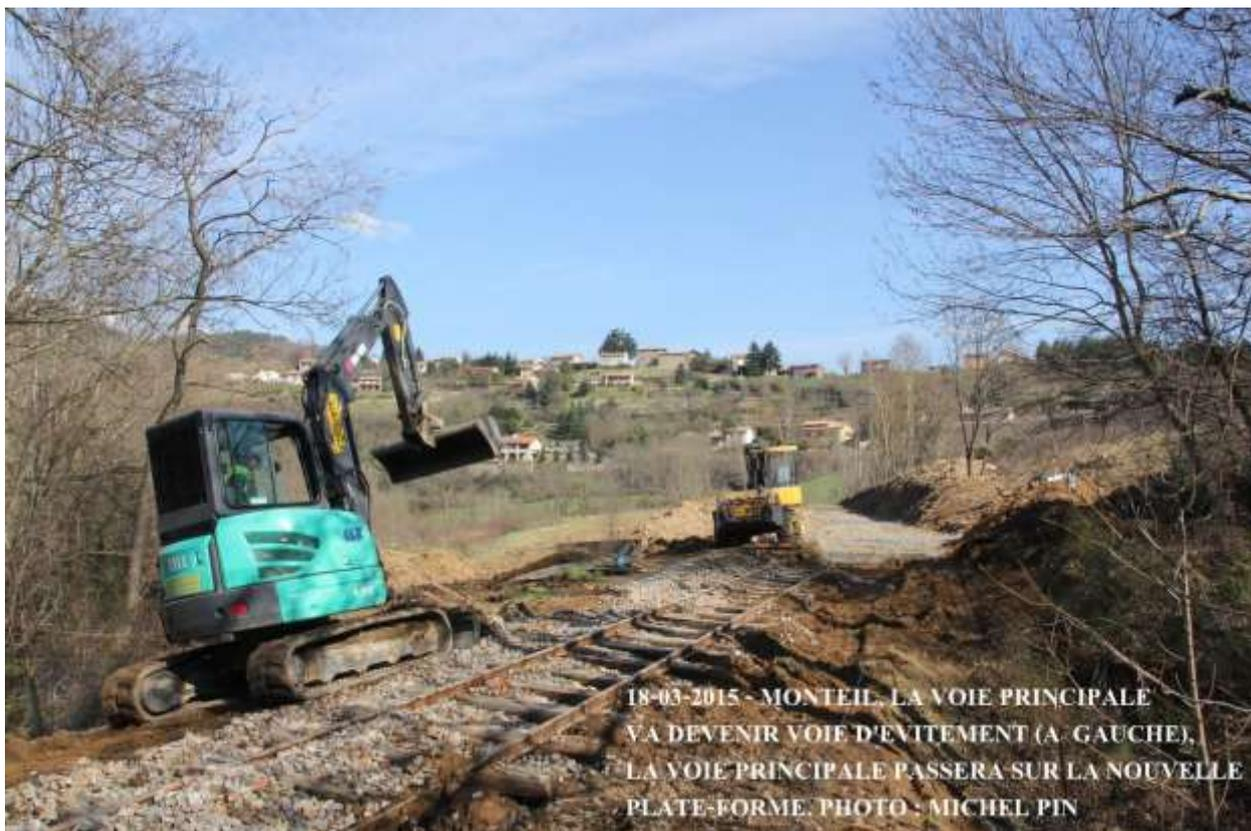
18-03-2015 - MONTEIL. LA VOIE PRINCIPALE VA DEVENIR VOIE D'EVITEMENT (A GAUCHE), LA VOIE PRINCIPALE PASSERA SUR LA NOUVELLE PLATE-FORME. PHOTO - MICHEL PIN
