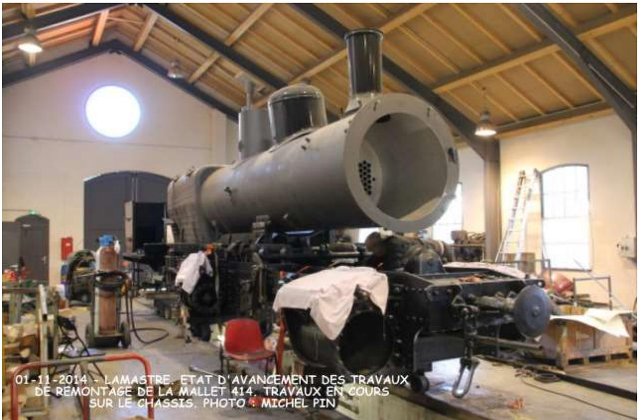
01-11-2014 - LAMASTRE. ETAT D'AVANCEMENT DES TRAVAUX DE REMONTAGE DE LA MALLET 414. TRAVAUX EN COURS SUR LE CHASSIS. PHOTO MICHEL PIN
